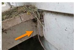
Ledger Board Flashing Missing
